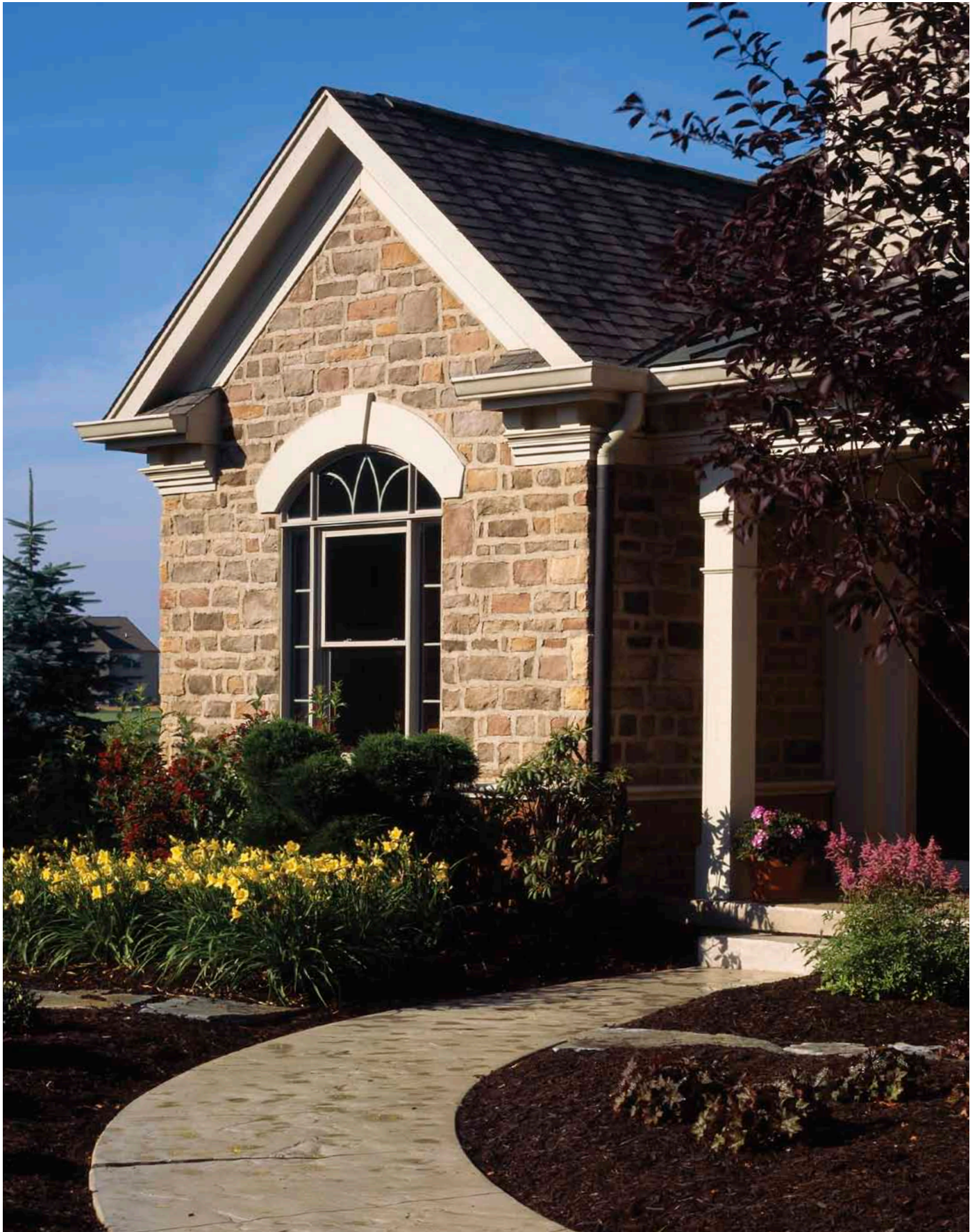
Bridgeport Limestone with an overgrout technique
