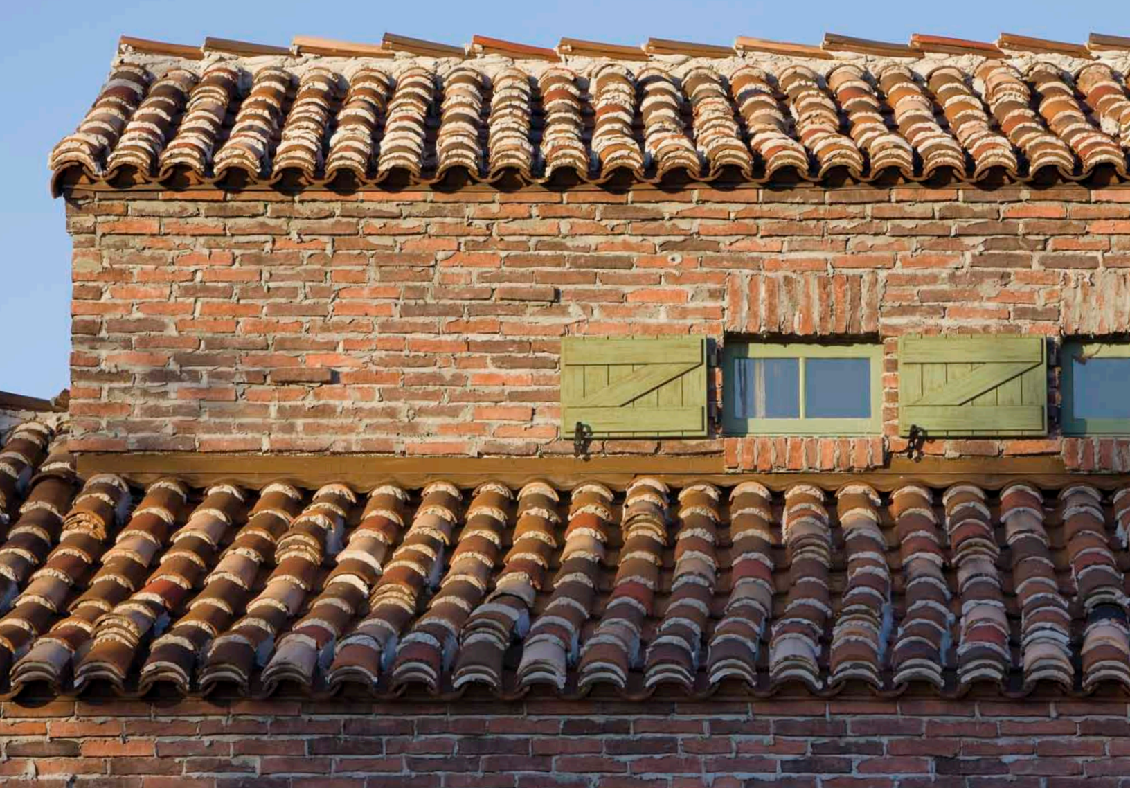
Bracciano RomaBrick with a weep joint grout technique
