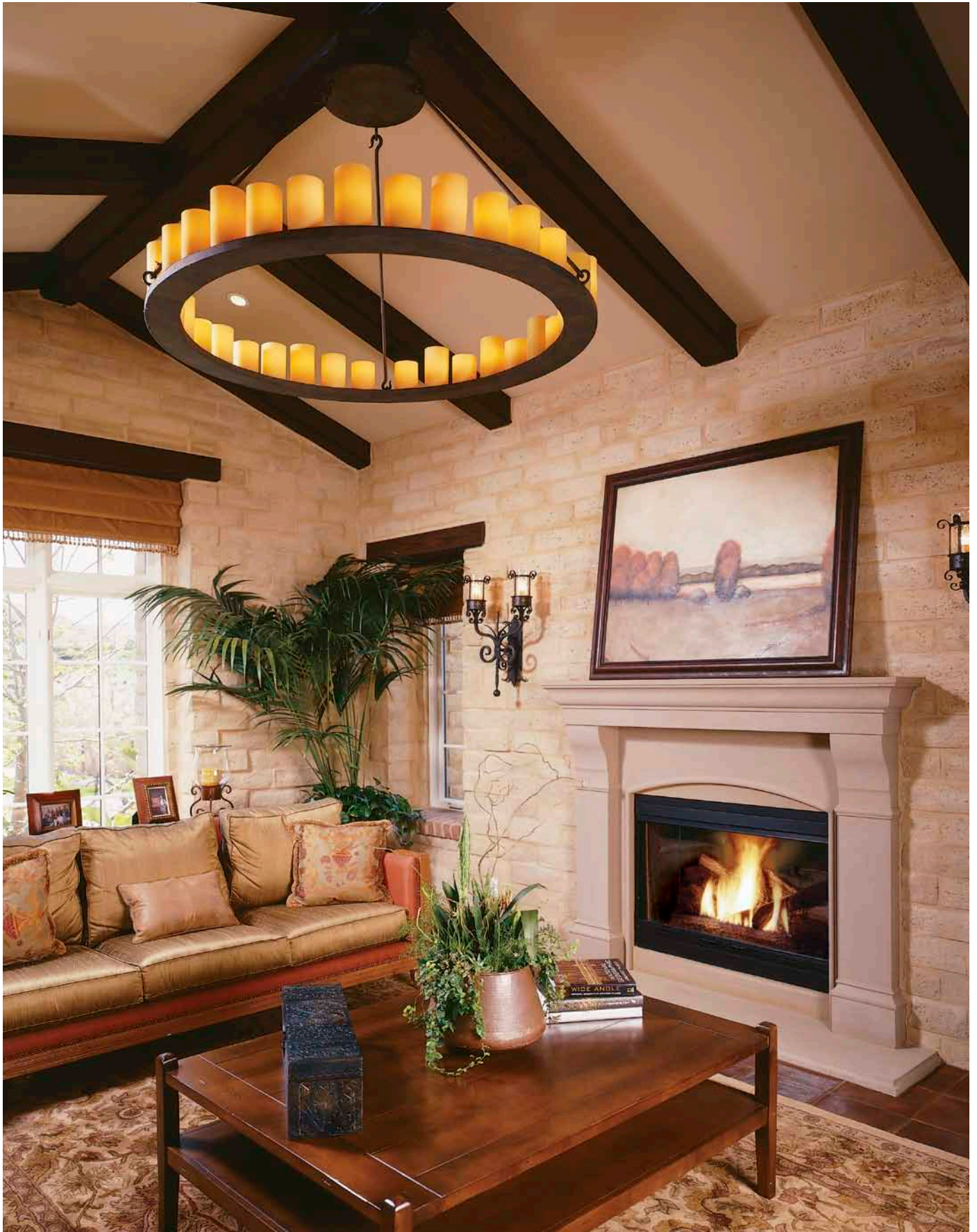
Solano Camino Adobe with an overgrout technique
