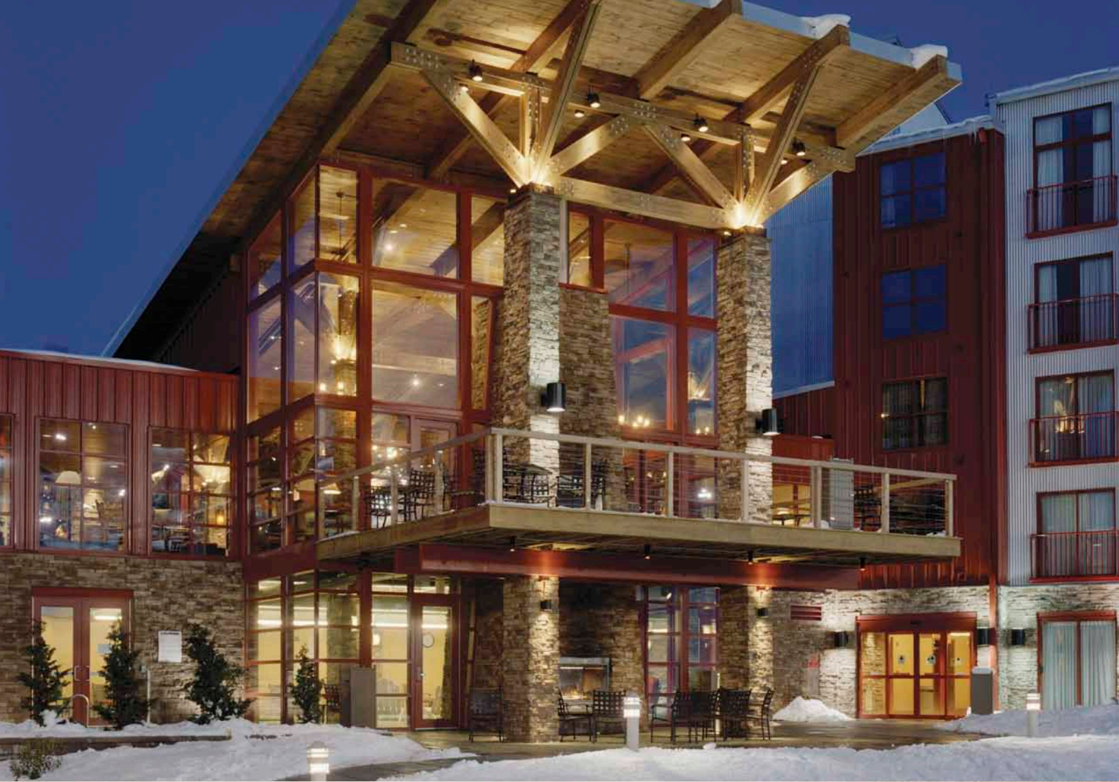
Charleston Mountain Ledge with a dry-stack grout technique
